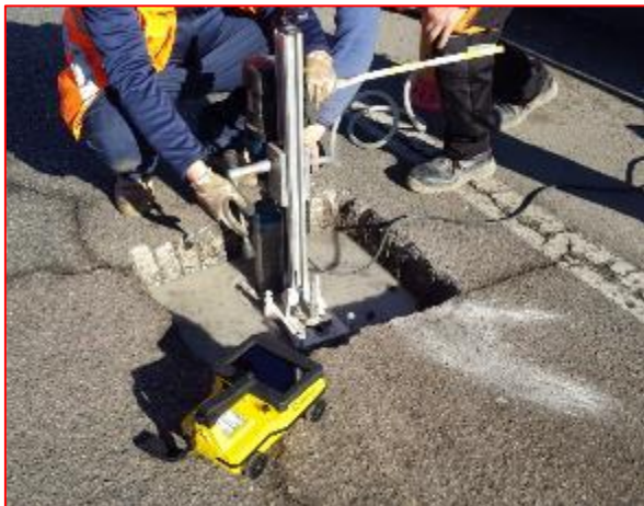
Reinforcement bars located
